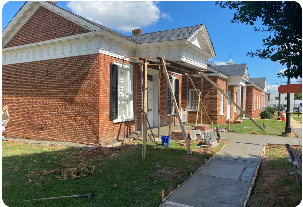
The Capital Improvement funding assists with critical projects, such as the restoration of Cumberland's historic court house facilities.
